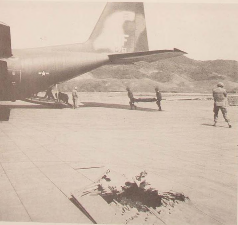
The impact of a 107mm or 122mm rocket caused this hole in the runway at Khe Sanh in 1967. Unlike most Soviet and some NATO fighters, USAF fighters cannot use grass strips and must have intact runways on which to take off and land.
